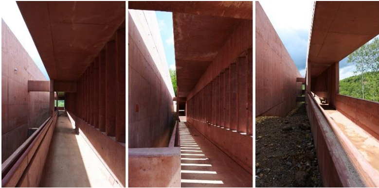
Figure 11-13: Views of the ramps around the protective building (courtesy by the Narmer Architecture Studio Budapest)
