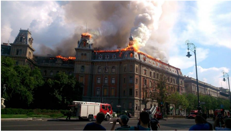
Figure 4: The burning roof on the Andrassy Avenue
